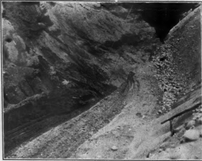
Bucket Excavating Mason's Sand
